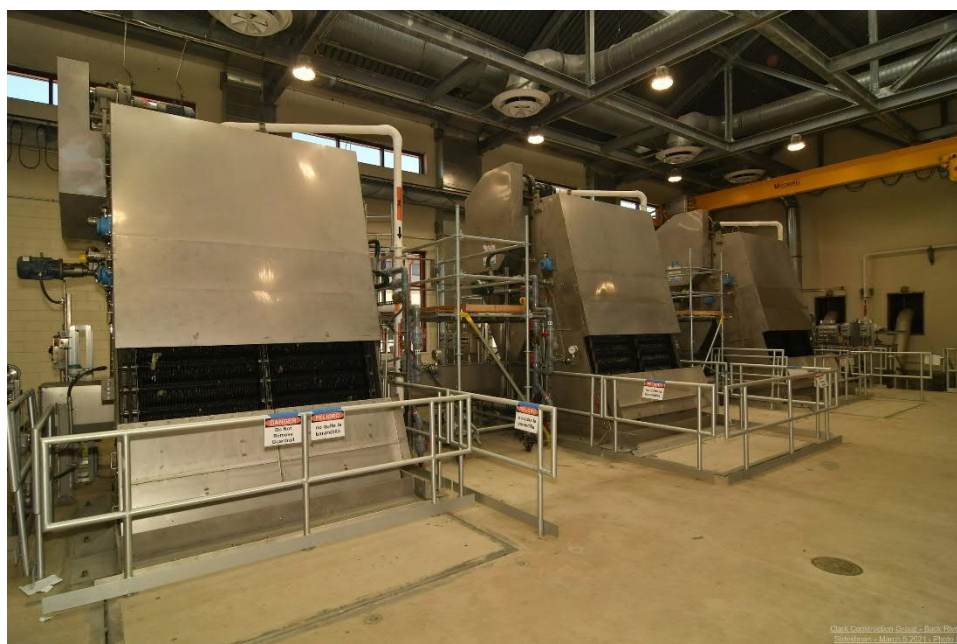
Back River WWTP Headworks Project – Fine Screen Facility; March 2021
